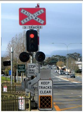
Figure 6.1 Traffic Signals Incorporated into an RX-5 Assembly
