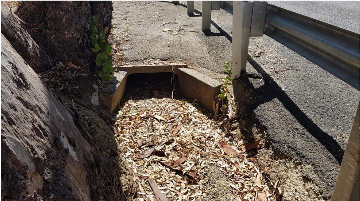
Figure 10: Culvert inlet Coral Avenue and Nairne Road intersection
