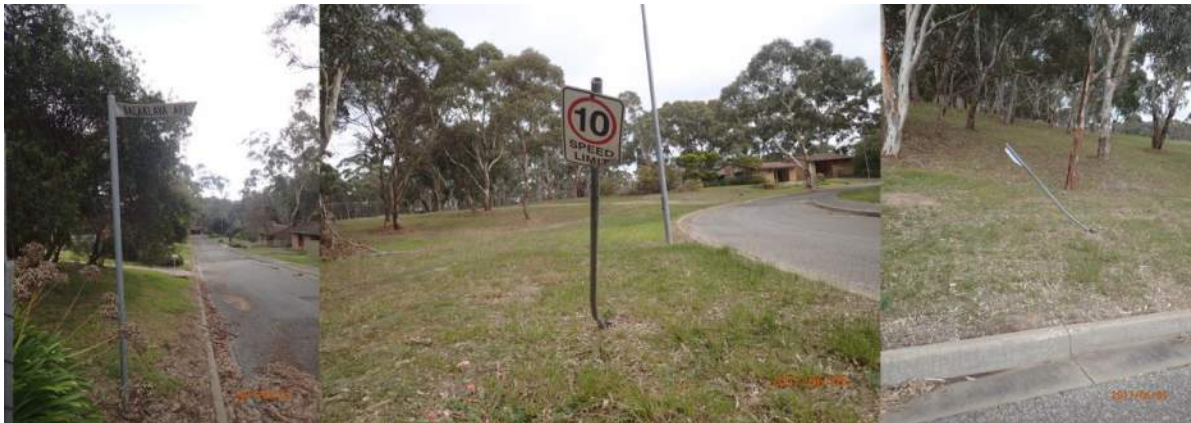
Figure 2.6 – Damaged Street Signs
