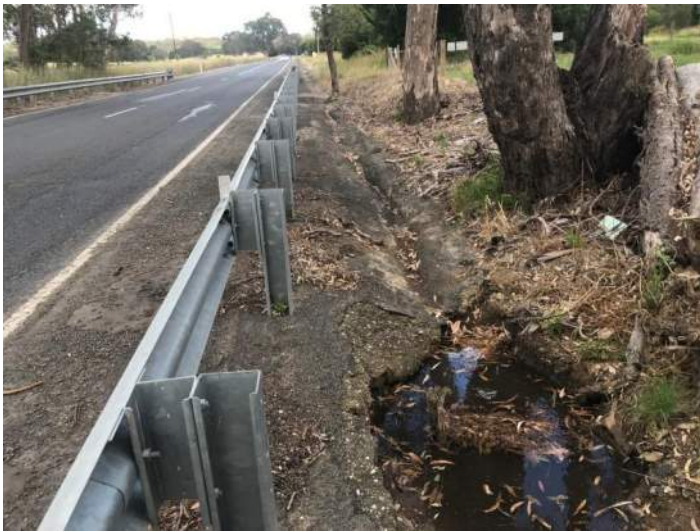
Figure 6: Roadside Swale (looking southeast)
