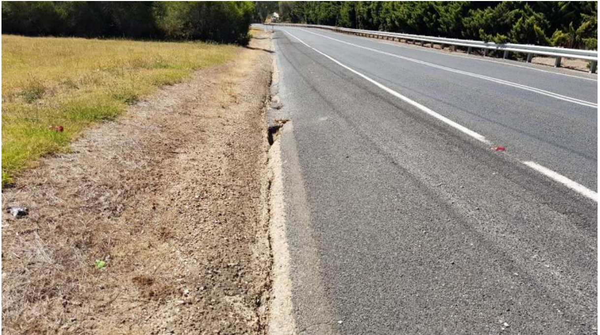
Figure 12: Roadside swale along Nairne Road
