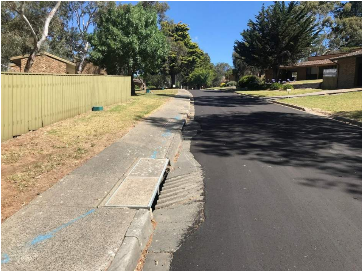
Figure 2: Site photo looking south up Caledonia Avenue (formerly Lucknow Ave).
