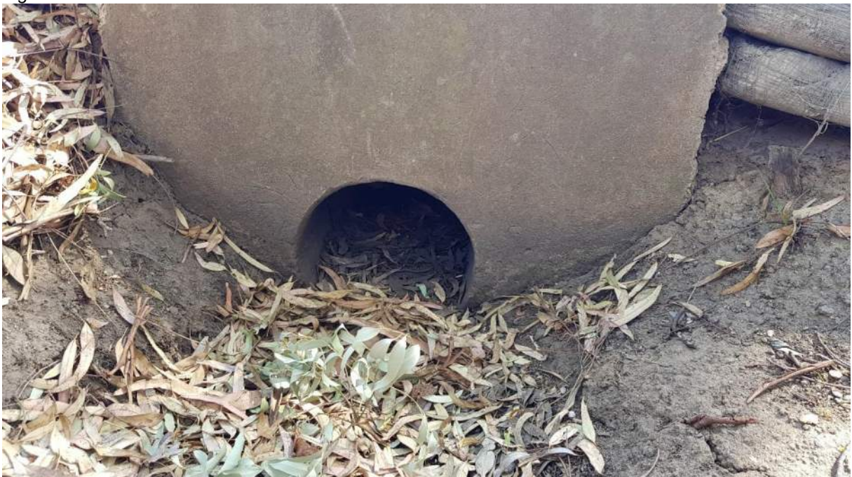
Figure 11: Culvert outlet Drummond Road and Nairne Road intersection
