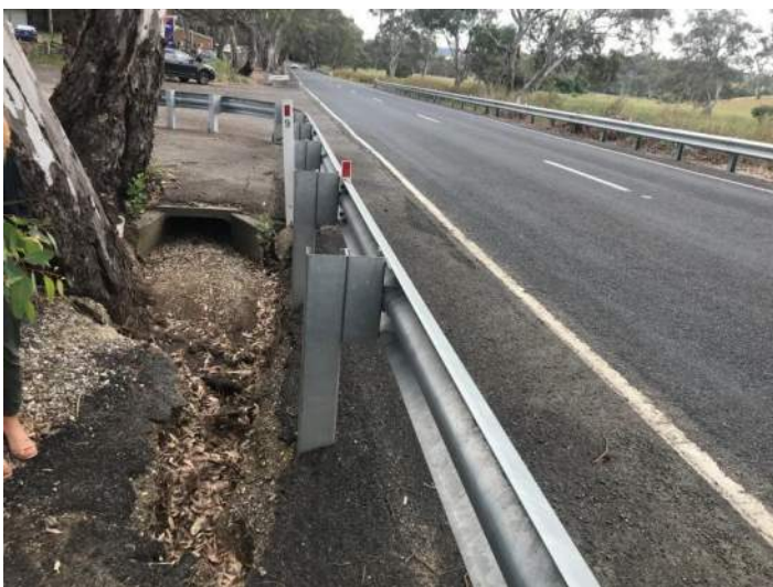
Figure 7: Headwall Inlet from Roadside Swale (looking northwest)
