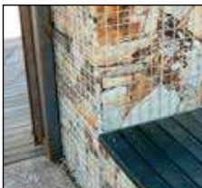
GABION CAGES CONTAINING LOCAL STONE
