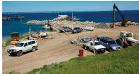
Informal parking, boat ramp access, heavy machinery and passenger ferry terminal access all conflict
