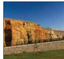
ROCK WITH NEW STONE (GABION WALLS)
