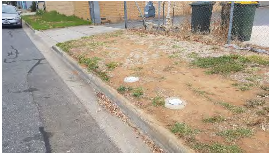
Photograph 1- View of GW01 and SV13 on the verge along Murray Street.
