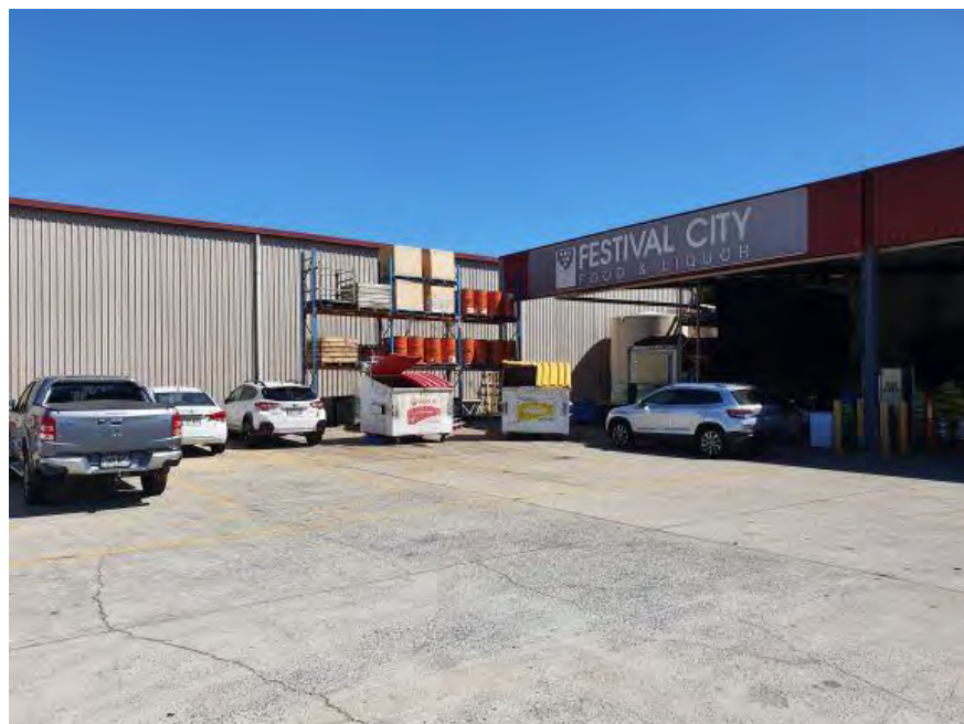
Photograph 6- View of the elevated storage of ethanol in 200 L steel drums, and concrete hardstand in the foreground.
