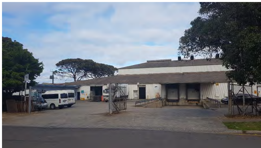
Photograph 15- View of the southern portion of Coast to Coast Services Pty Ltd.
