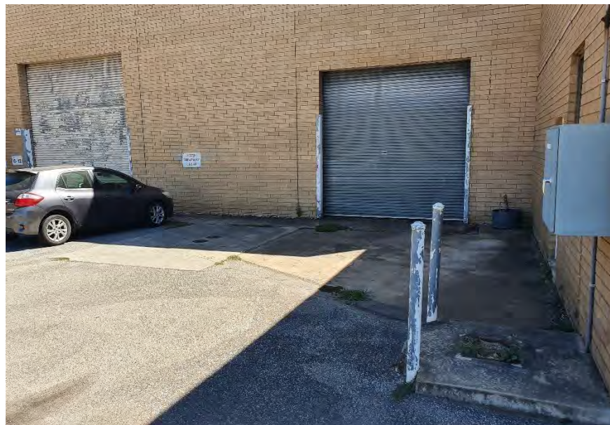
Photograph 4- View of the suspected UST with surface covers of the dip and fill points visible. Former bowser plinth is visible in the front right of the photo.
