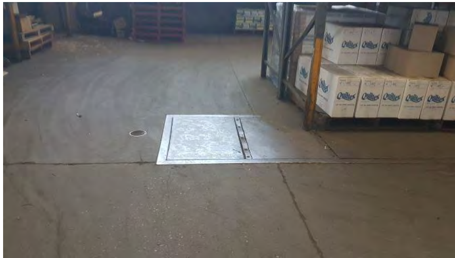
Photograph 3- View of suspected grease arrestor with inspection cover.
