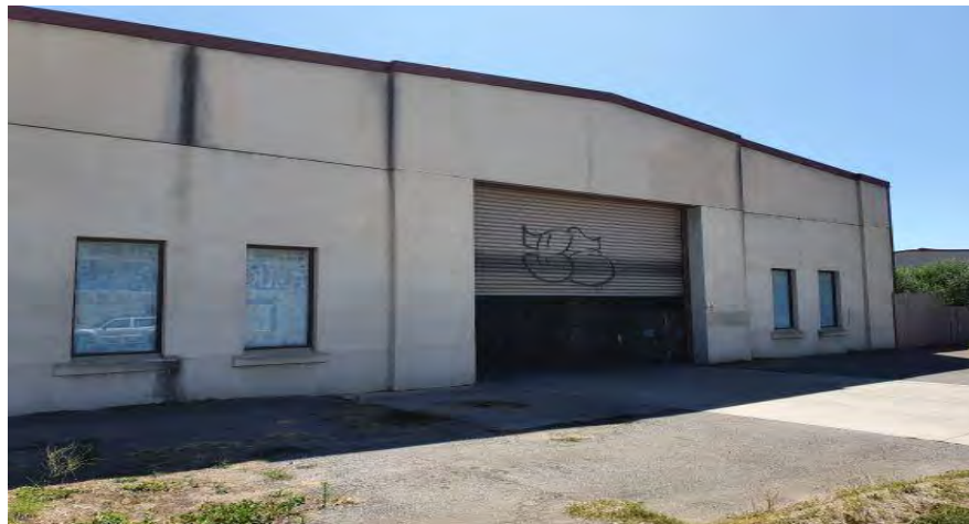
Photograph 5- View of the warehouse May Street entrance. The suspected UST was located to the left (south) of the roller door.
