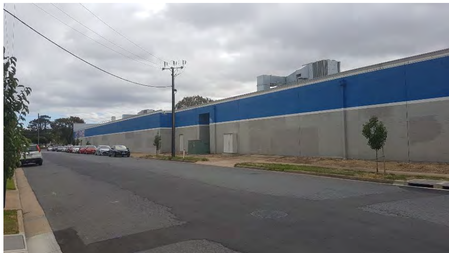
Photograph 9- View looking north of the Spotlight building along May Street.
