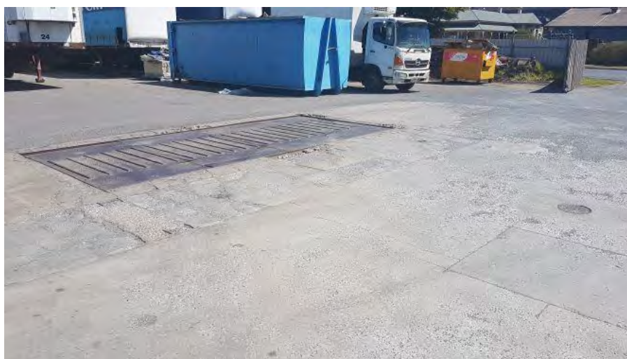
Photograph 2- View of the large suspected service pit and UST.
