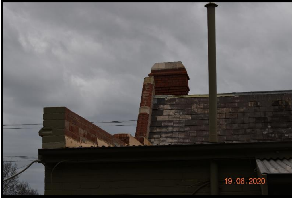
Photograph 13 – Parapet wall. Note flashing.
