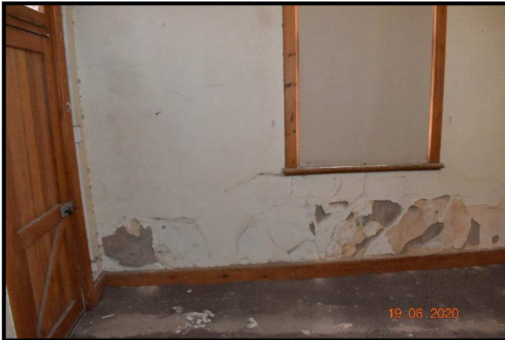
Photograph 4 – Living G4. Note deterioration of the stone masonry.
