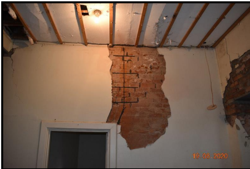
Photograph 8 – Note retrofitted movement joints and propping of the ceiling lining
