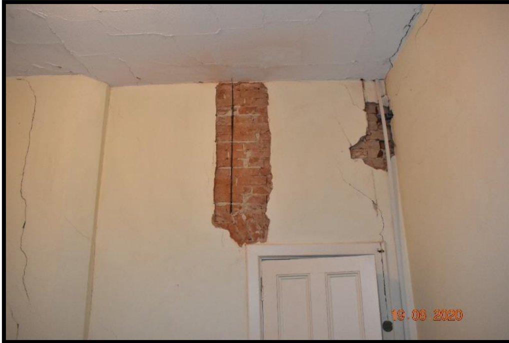
Photograph 9 – Bedroom G3. Note wall cracking and retrofitted movement joints
