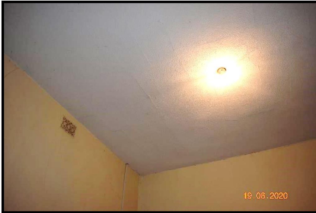
Photograph 7 – Bedroom G3. Note slight cracks in ceiling lining
