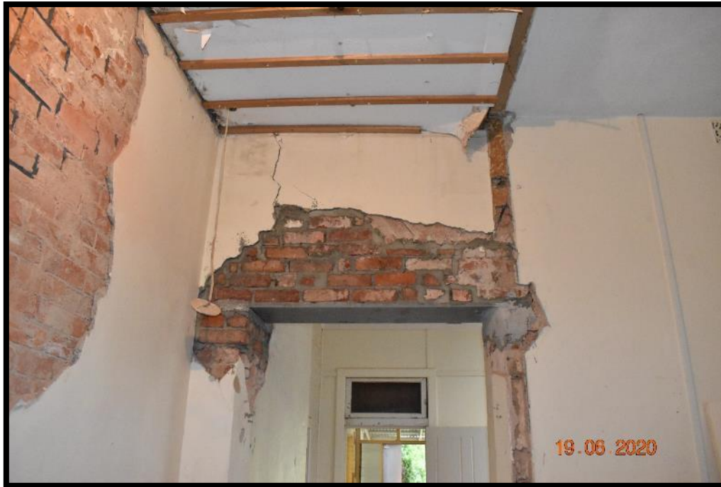
Photograph 5 – Hallway G1. Deteriorated ceiling lining and wall cracking.
