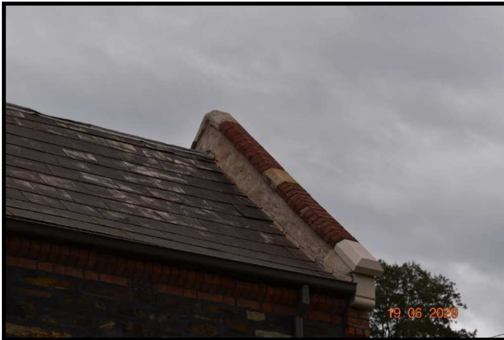
Photograph 12 – Parapet wall. Note flashing.
