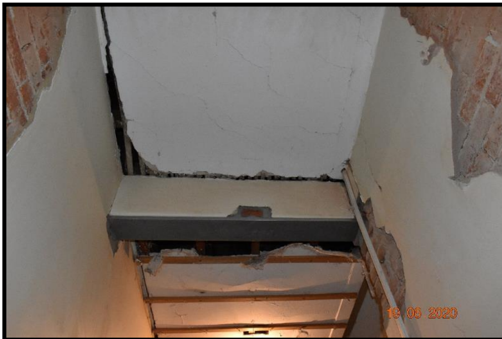
Photograph 6 – Hallway G1. Deteriorated ceiling lining and wall cracking.
