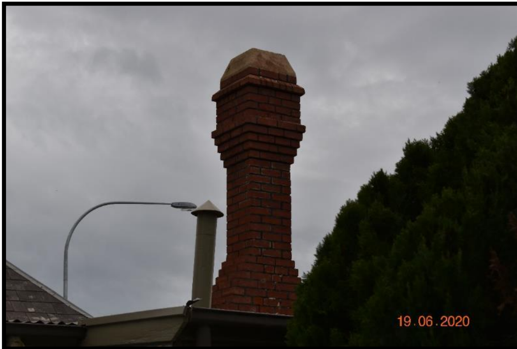
Photograph 10 – Chimney. Note height of chimney extending above the roof level.
