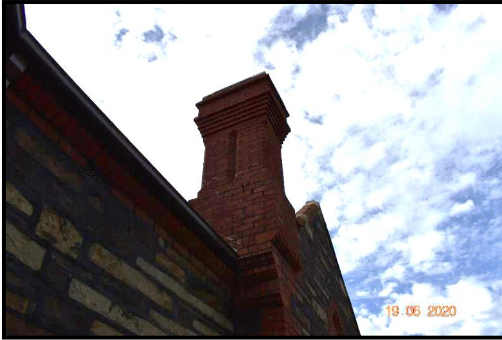
Photograph 11 – Chimney. Note height of chimney extending above the roof level.
