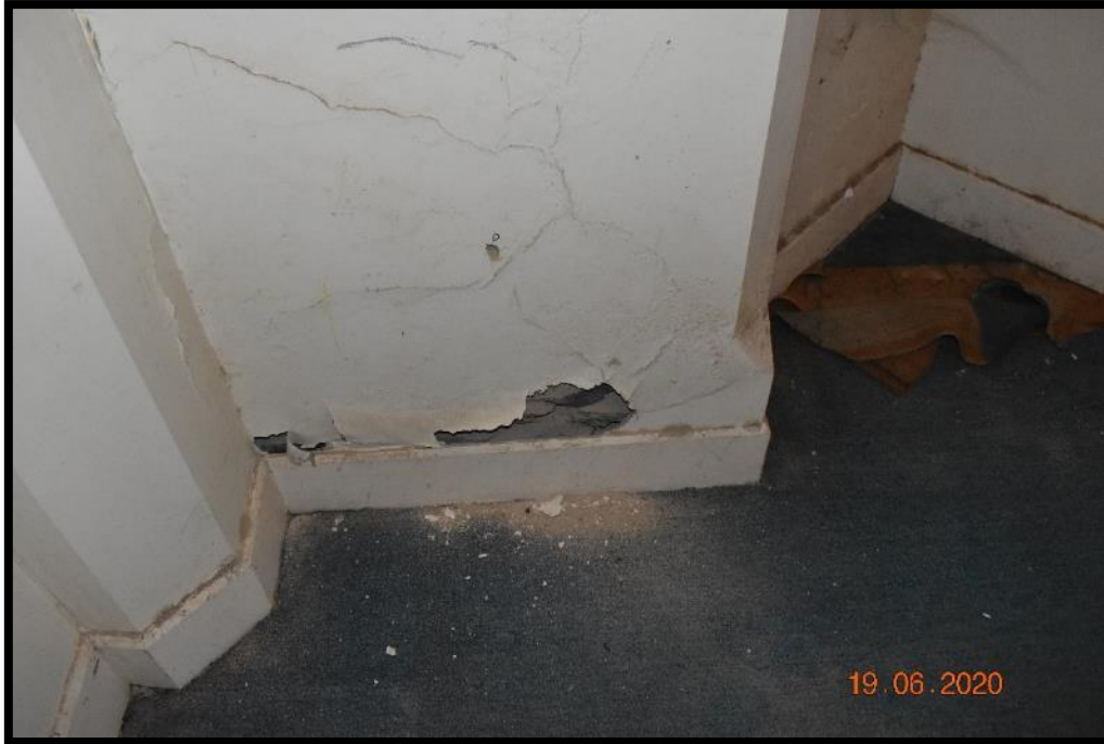
Photograph 3 – Bedroom G2. Note deterioration of the stone masonry including loss of cross-sectional area.
