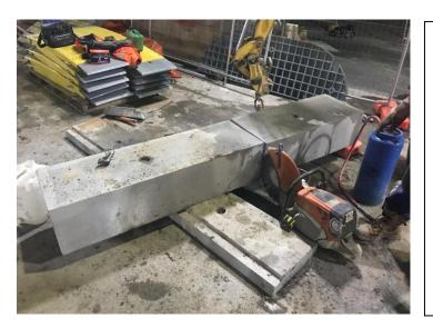
A worker was recently injured when the quick cut saw he was using to cut a concrete box culvert jammed and kicked back, injuring his upper arm.
