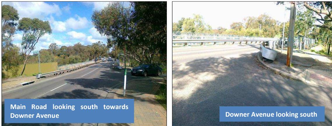
Figure 7.1.3.4 - Main Road/ Downer Avenue
