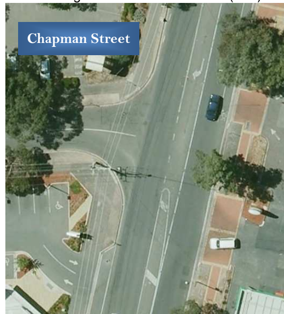
Figure 7.1.10.1 - Aerial of Junction (2014)
