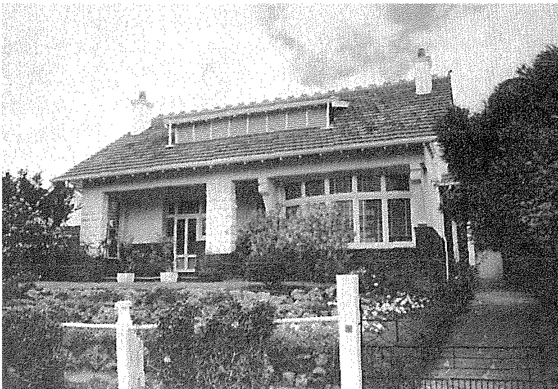
Glenelg Heritage Survey (Stage One) p161
