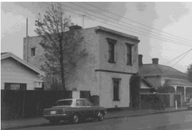
34 Waterloo Street, 1980 - PH-GL-1183 Holdfast Bay History Collection
