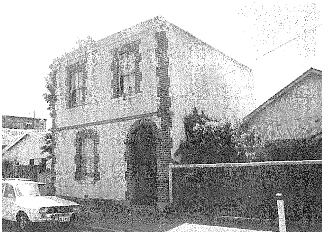
Glenelg Heritage Survey (Stage One) p132
