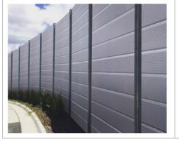
The panels are constructed from a high-density PET core and a pre-coloured, perforated aluminium outer skin. Sound waves penetrate the perforated face of the panel and are absorbed within the core material, resulting in high sound-insulation performance. The products are effective for noise intensive environments, such as noise and rail corridors, as well as businesses that make extensive use of loading docks, heavy machinery, or large-scale generators.
