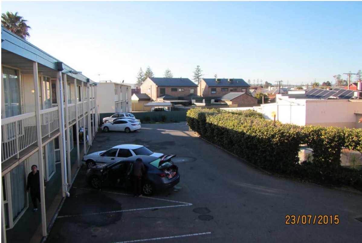
Photograph 9: View east across sealed carpark area from first floor of hotel.
