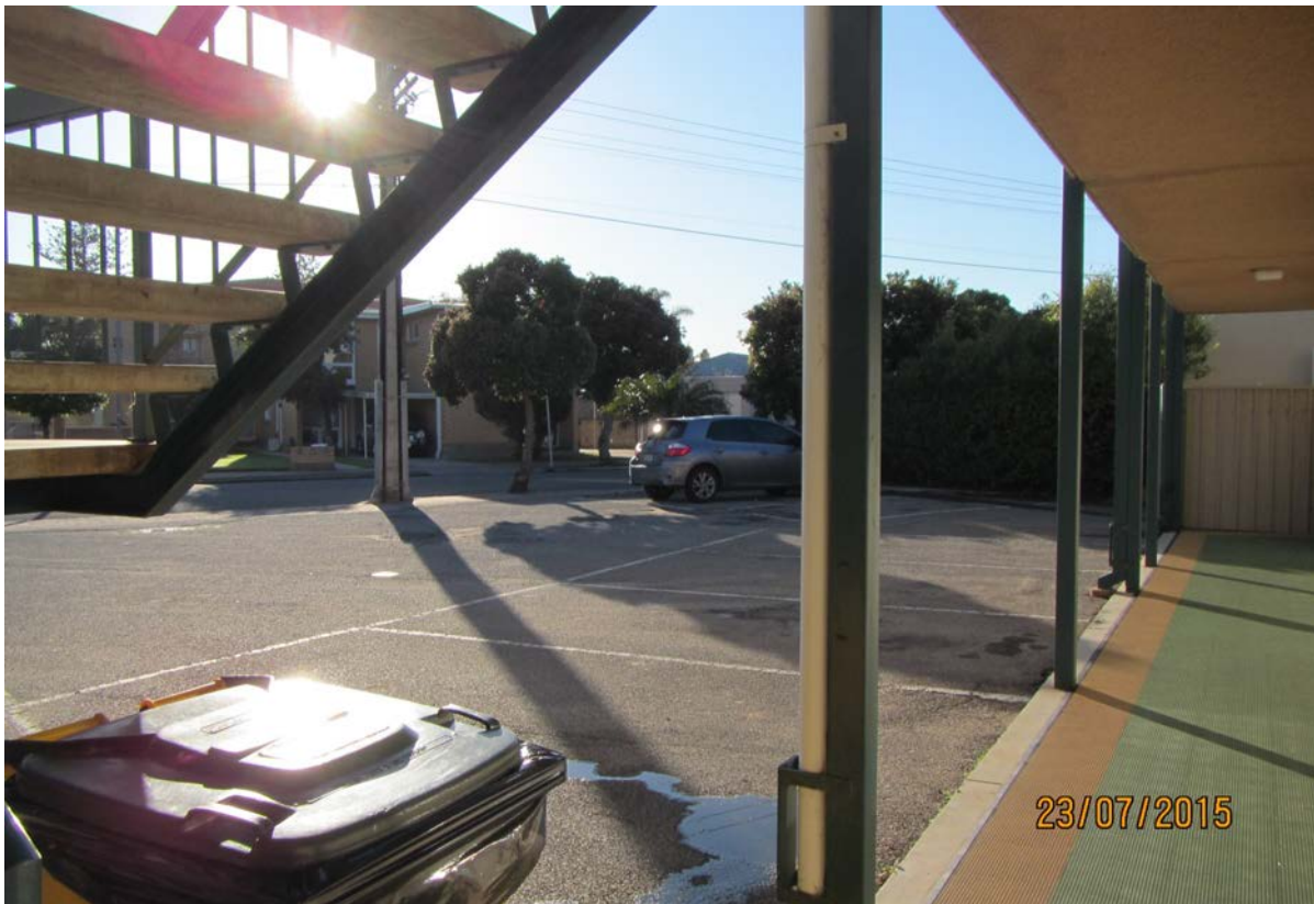
Photograph 8: View north east of adjacent residential properties across northern most carpark.
