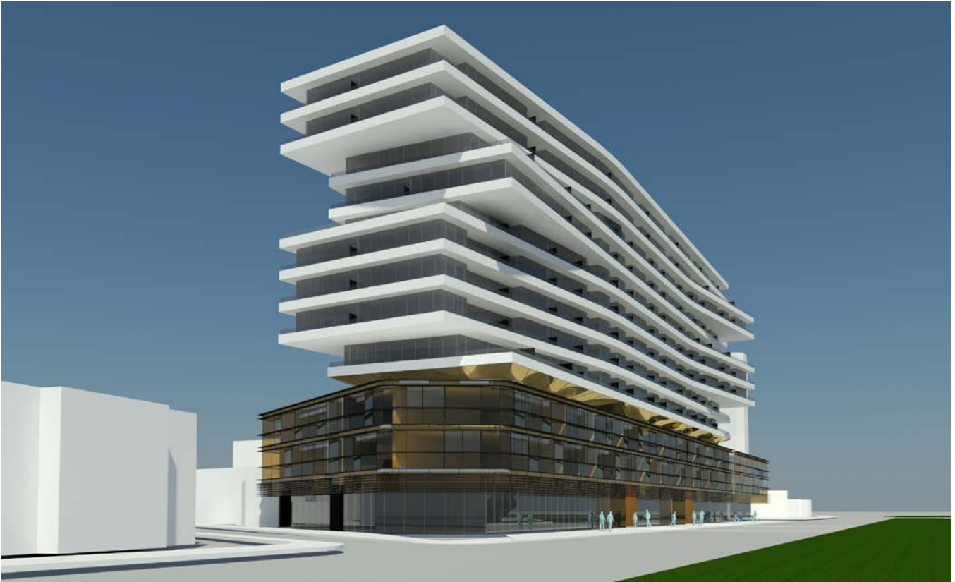
Cantilevered floor plates
