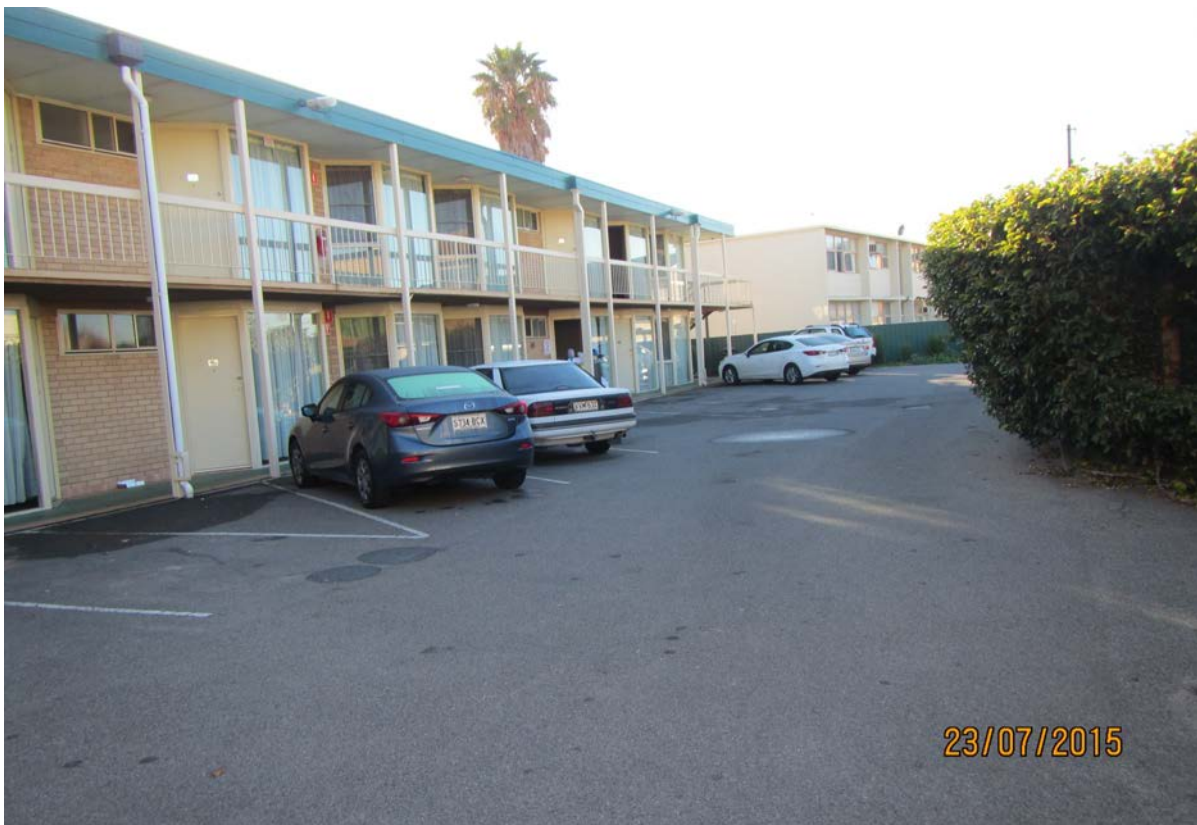
Photograph 4: View east across sealed carpark area.
