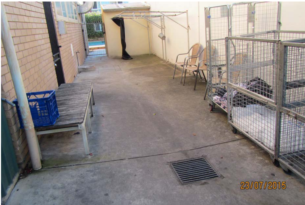
Photograph 1: View north through service road in the central portion of site showing stormwater drainage.
