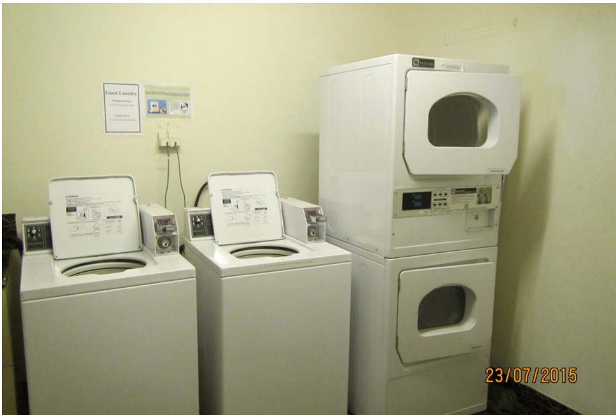
Photograph 11: Tenant laundry facilities.
