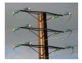
Typical disk insulator of a 33kV powerlines (3 disks)
