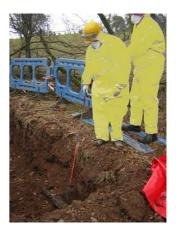
Pipes should be thoroughly wetted before work and during the work. This team had a pumpable spray, but other methods are acceptable (e.g. watering can, pouring from a bucket, etc). Cut only with hand tools, or break out with hammer after wetting.
