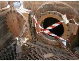
Left: Manway into a digester with mechanical guard fitted. Right: Manway entry for the digester without scaffolding (tape placed by emergency response team).
