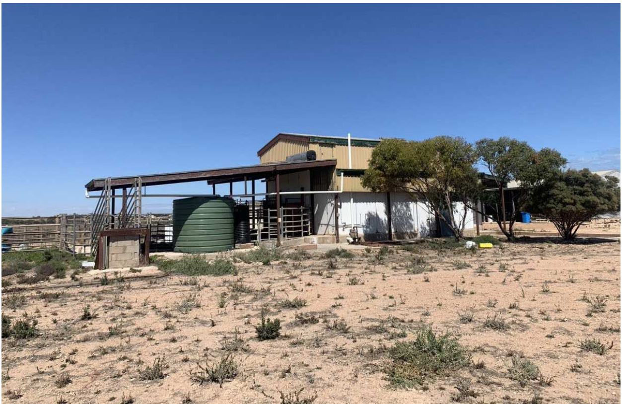
Photograph 2: Views to the east of the abattoir and sheds beyond.
