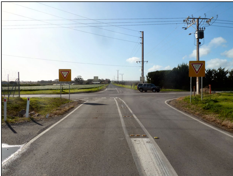
Figure 9: Narrow painted median with RRPMS
