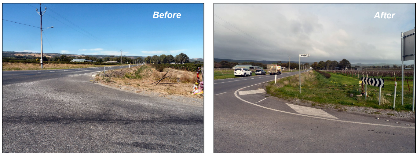
Figures 8a & 8b: Before & After corner treatments installed
