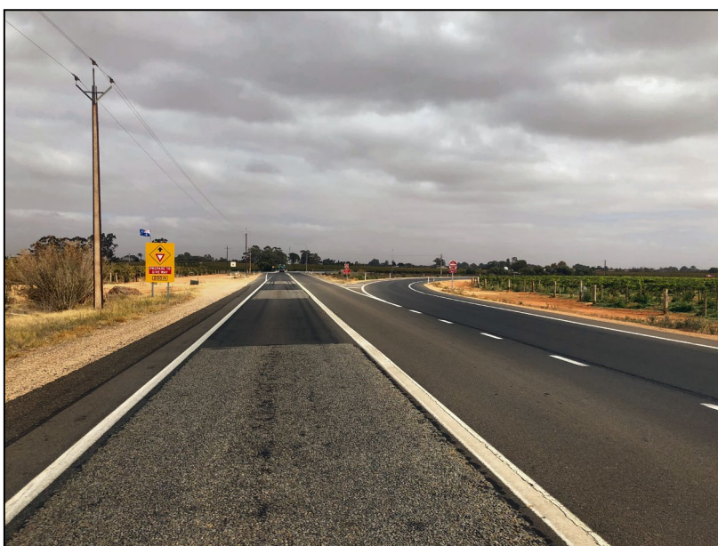
Figure 10: Rumble strips on approach to intersection
