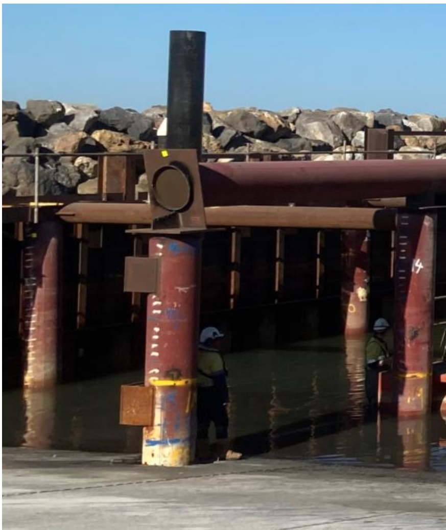
Returning water to the ramp area - 29 December 2021
