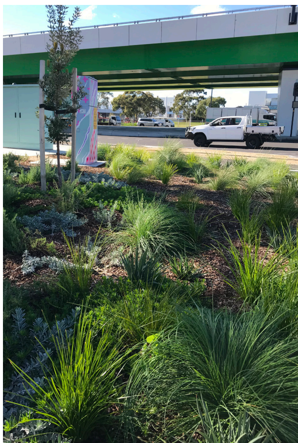
North South Corridor (Regency to Pym project) Diverse understory planting at Regency Road-South Road intersection
