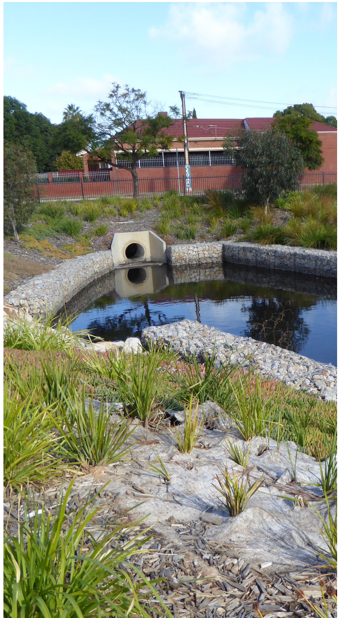
North South Corridor (Torrens to Torrens project) Cedar Ave, Croydon, Gross pollutant and sediment basin
