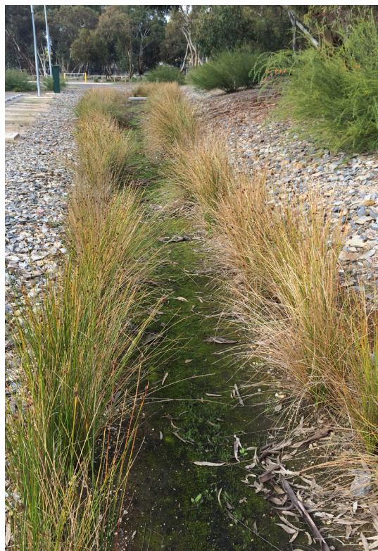
Klemzig Interchange Western carpark – rock lined biofiltration swale.
