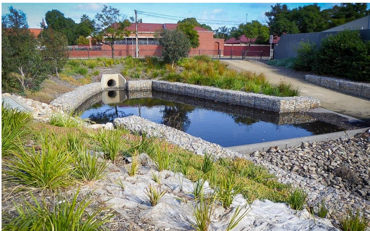
Gross pollutant and sediment basin, North South Corridor (Cedar Avenue).
