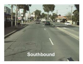
■ **Section 5**: The Crescent to Jetty Road (Brighton) – this section consists of 2 traffic lanes in both the northbound and southbound directions within a typical road width of 19m.
