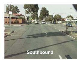
■ **Section 4**: Oaklands Road to The Crescent – this section consists of 2 traffic lanes in both the northbound and southbound directions within a typical road width of 19m.
