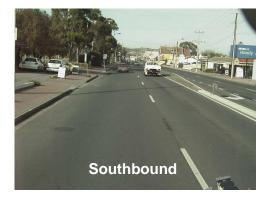
■ **Section 6**: Jetty Road (Brighton) to Sturt Road – this section consists of 2 traffic lanes in both the northbound and southbound directions within a typical road width of 19m.
