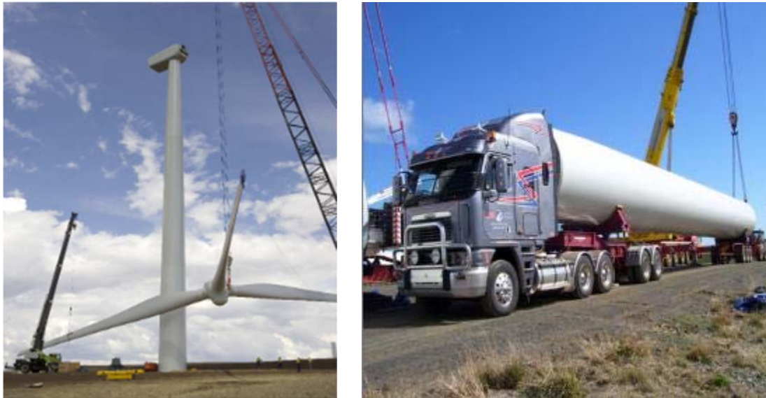
Figure 32 An example of a cranes employed to erect a wind turbine
