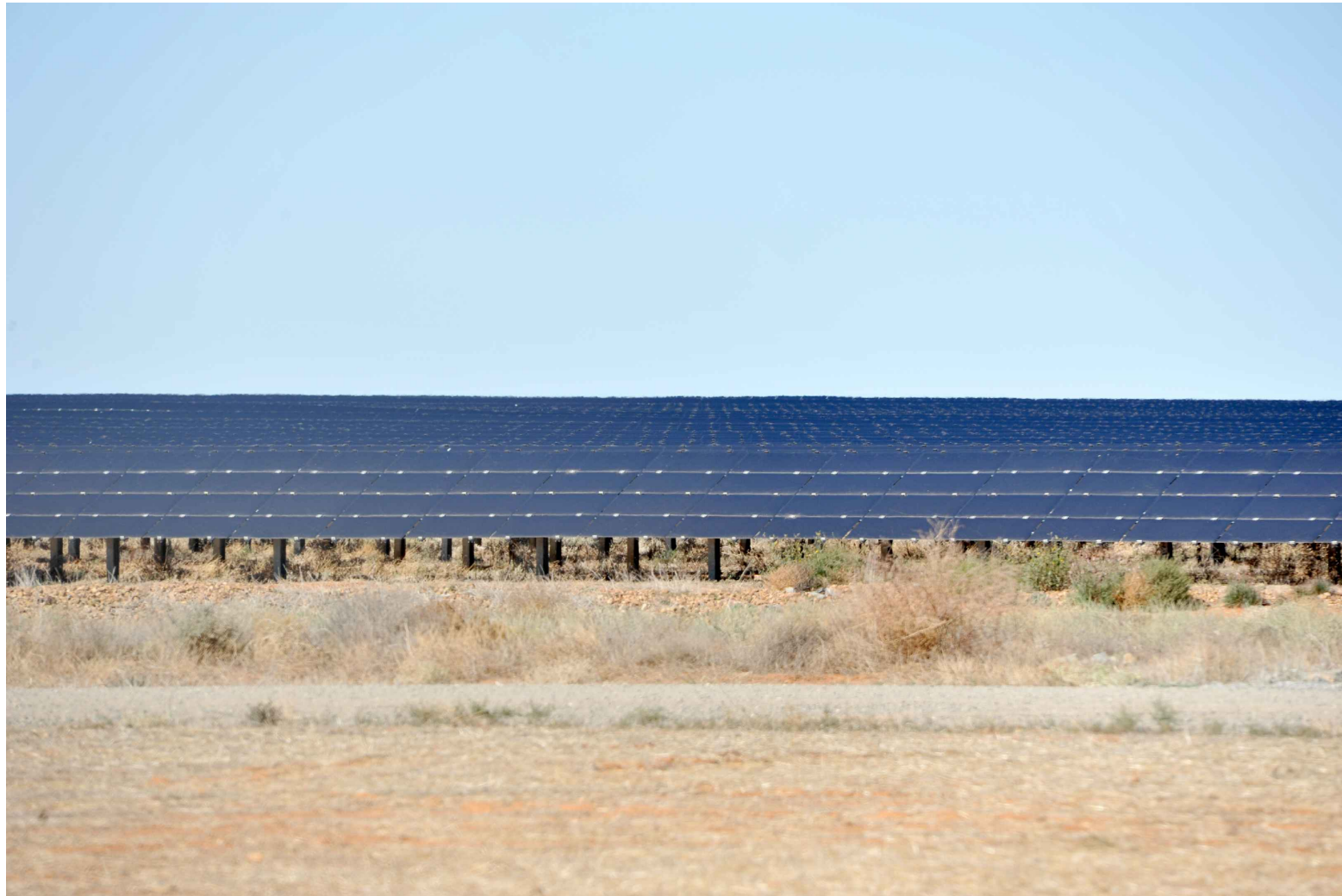
Plate 5 - Typical view toward photo voltaic panel face (single axis track)
