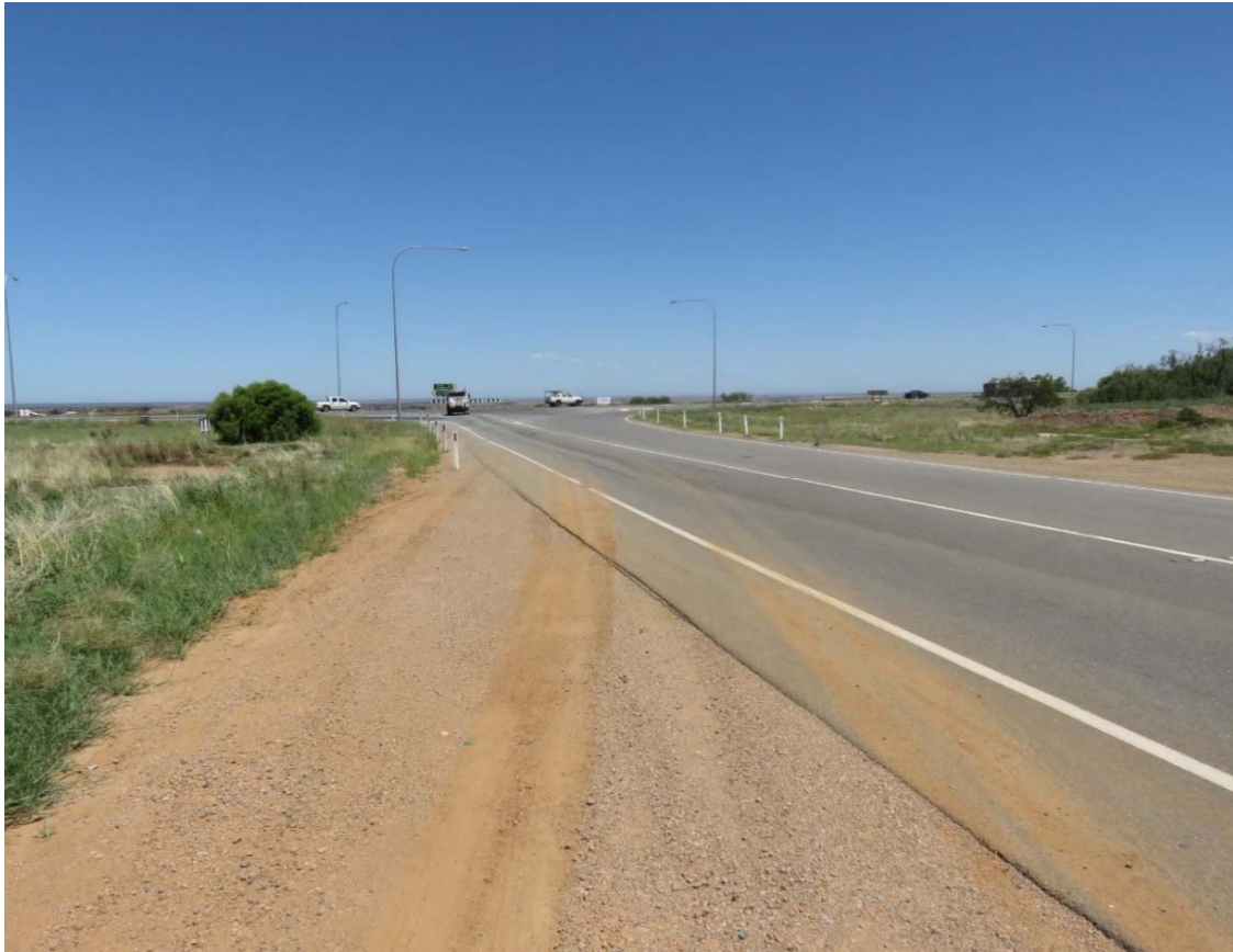
Figure 18 Wilkins Highway and Augusta Highway intersection looking west
