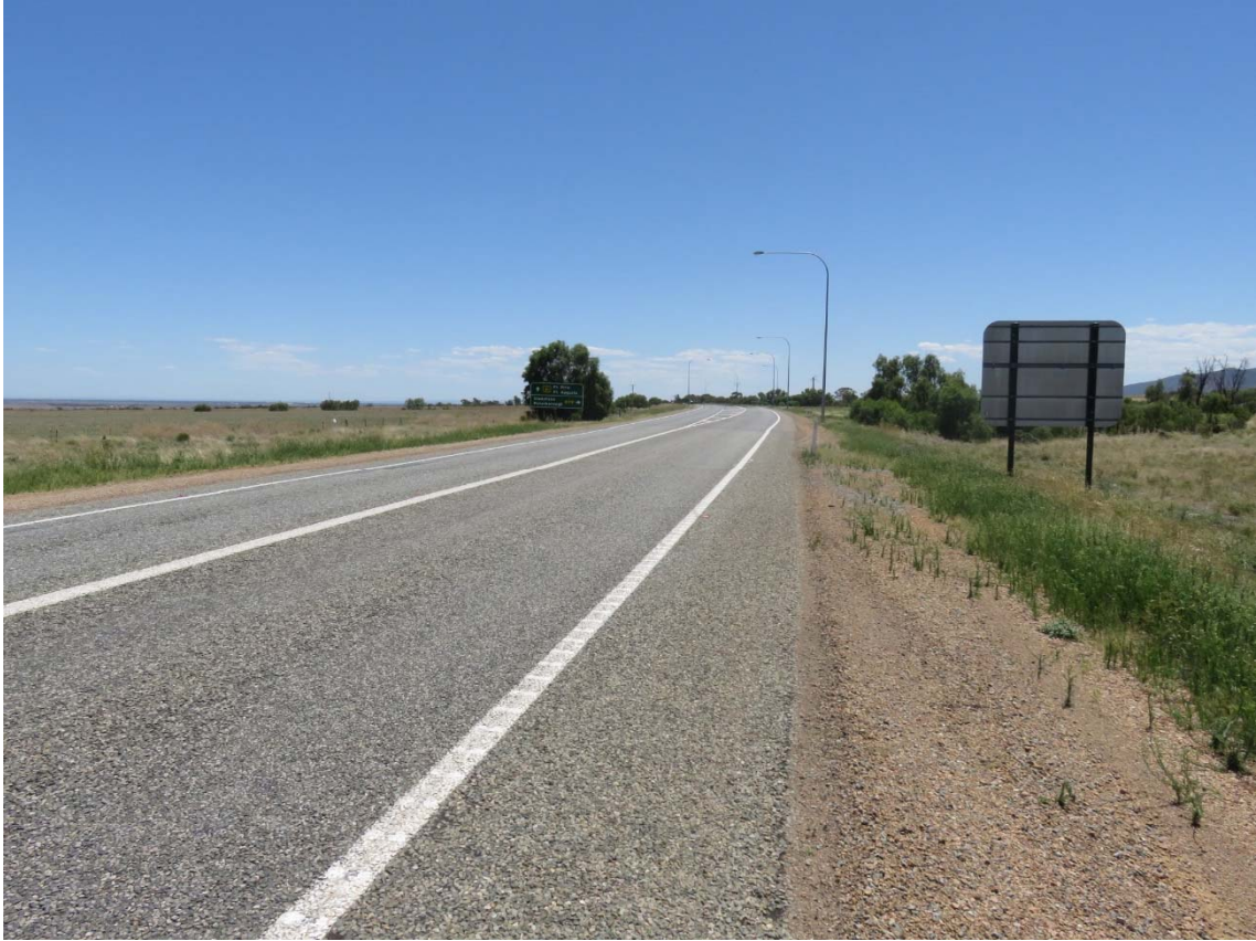
Figure 19 Augusta Highway on approach to Wilkins Highway looking north
