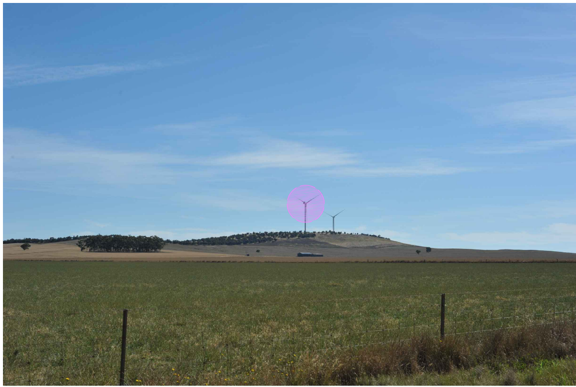
Maroona Wind Farm - View distance 2 km
