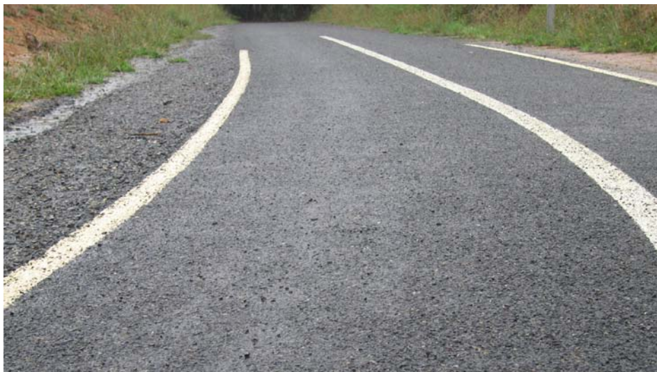
Figure 3.1 Spray sealed bikeway
