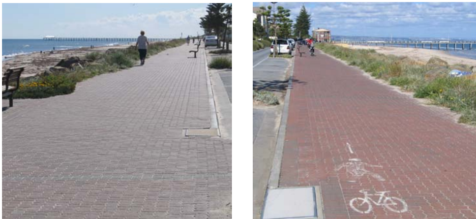
Figure 6.1: Concrete block paver shared bikeway
