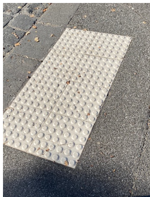
Photo: Pram crossing, Parkville
