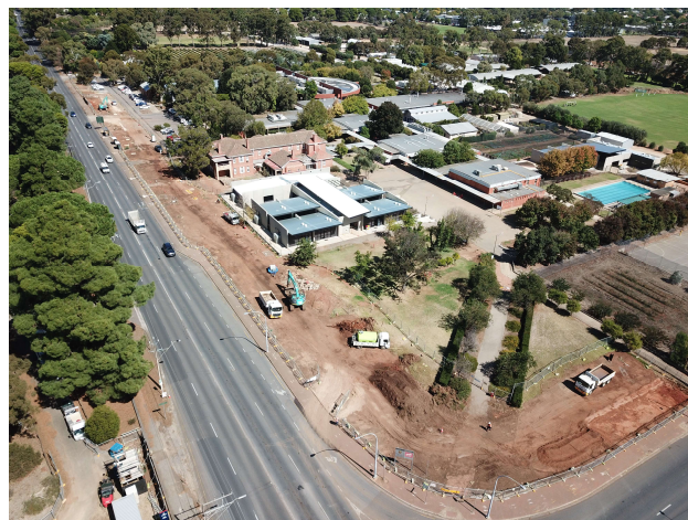
Image showing progress of work at the intersection in mid-April 2022.
