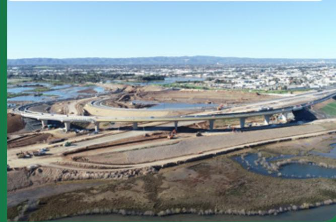
**FAST FACT** Approximately 1,100 concrete piles installed across the project
