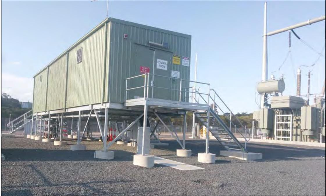
Figure 4-6: Example of a Typical Switch Room
