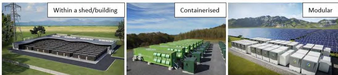
Figure 4-4: Examples of Utility Scale Battery Technology Options
