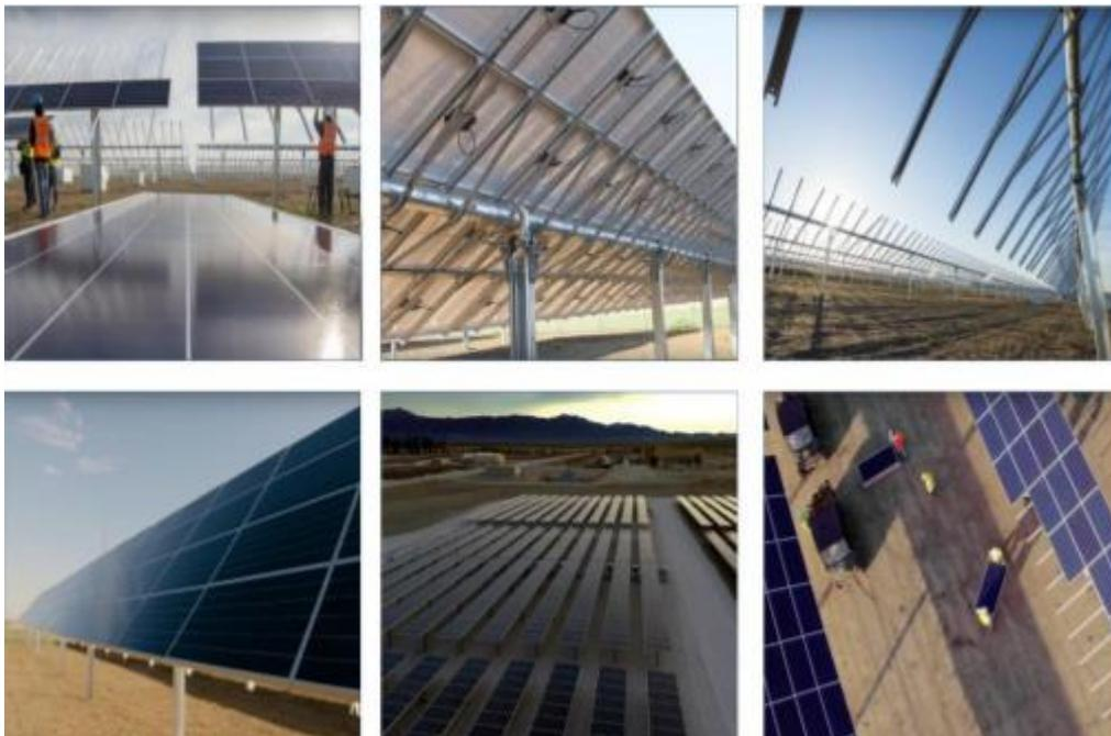
Figure 1: examples of typical single axis tracking solar modules
