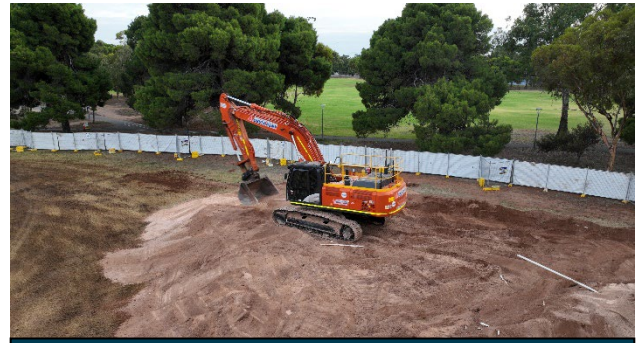
Excavator working on site
