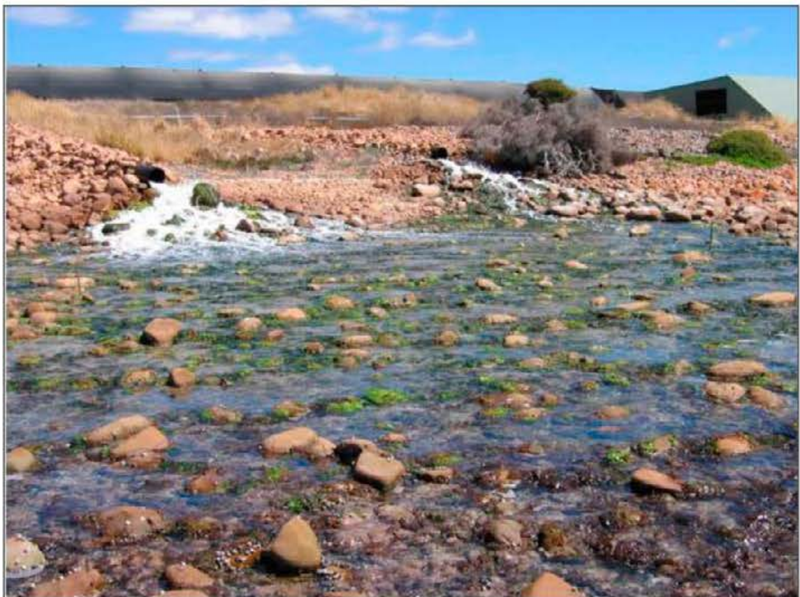
Figure 2-8 Outfall pipes discharging land-based abalone farm seawater to intertidal shoreline at Smith Bay (source: Tanner & Bryars, 2007)
