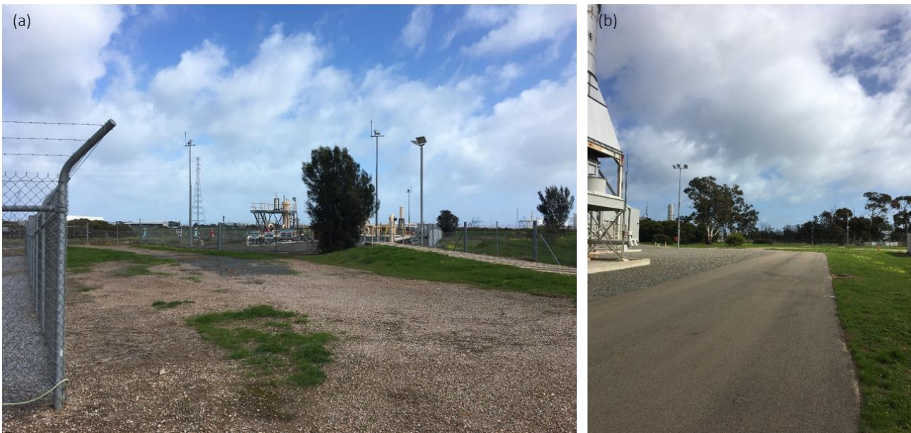
Figure 6: Onshore infrastructure location (a) shallow culvert and (b) vaporisers
