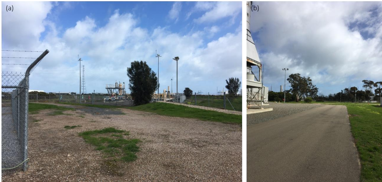
Figure 16: Onshore infrastructure location (a) shallow culvert and (b) vaporisers
