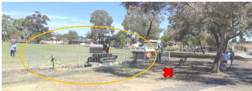
900mm _ Crowd Control Barriers used for deep excavation on school oval
