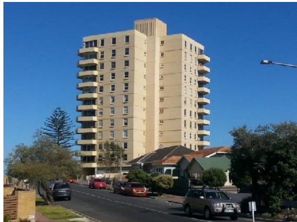
From the east – residences in the foreground
