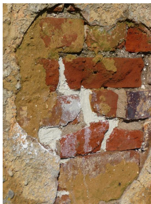
Repointing of a brick wall using lime mortar
