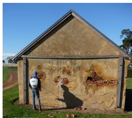
Pre-wetting of wall to prevent suction.
