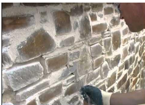
A stone wall being repointed using lime mortar.
