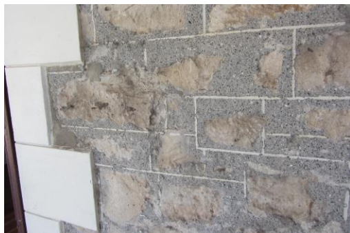
Original white lining on limestone wall.
