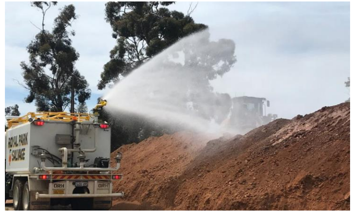
Watering stockpiles to minimise dust
