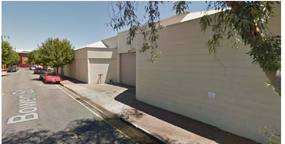
Image 5. Subject Site's warehousing interface with Bowen Street. Source: Google Maps
