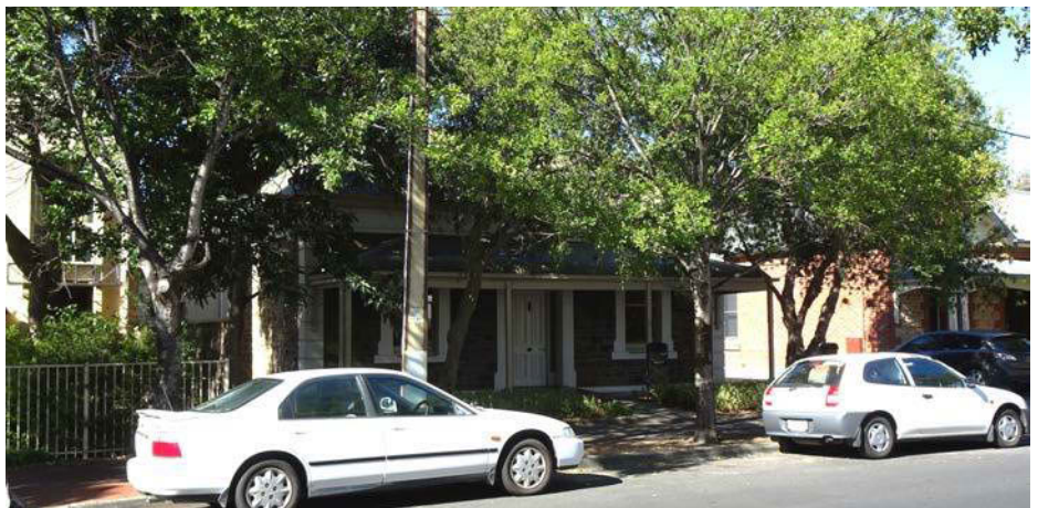
Image 24. Local Heritage place, 21 High Street Kensington
