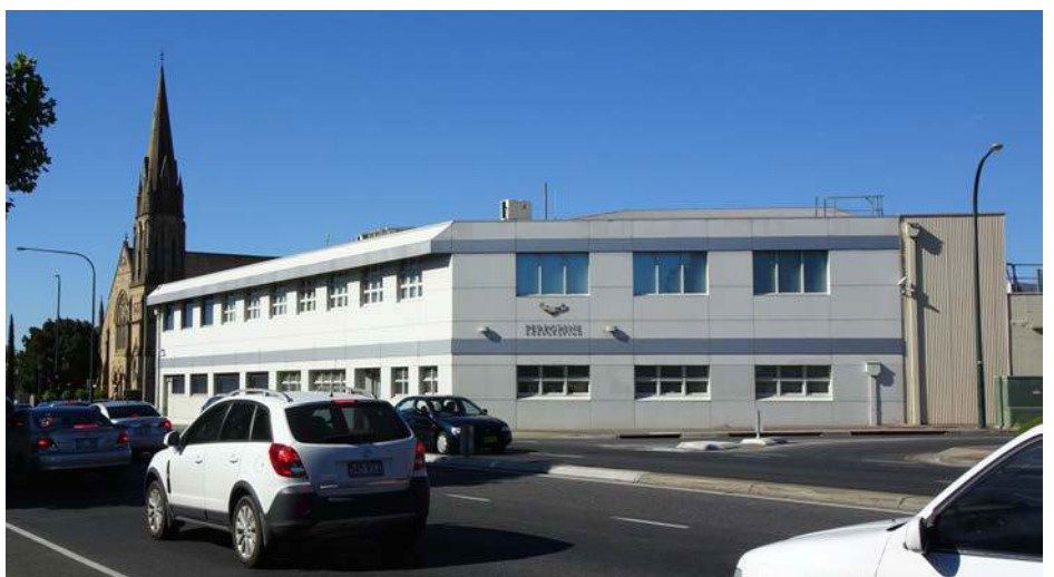
Image 3. Subject Site interface with Portrush Road and High Street intersection
