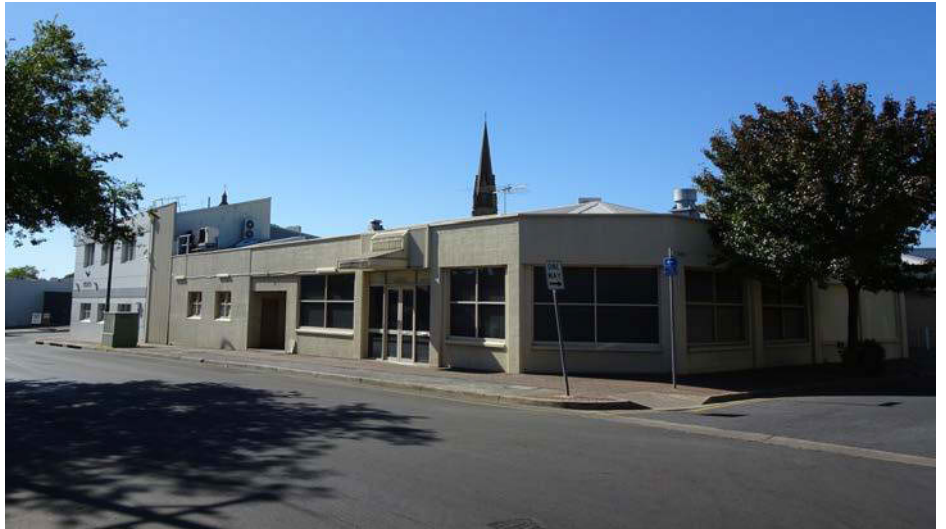
Image 4. Subject Site interface with Portrush Road and High Street intersection
