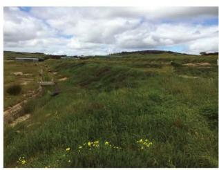
Photograph 14: View looking east at cut and levelled platforms. Drains with pipes discharging into them can be seen
