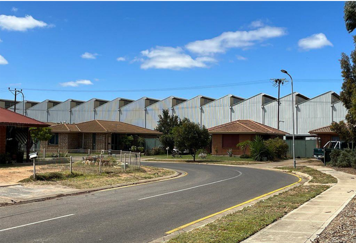
Photograph 2: Arthur Street looking east.
